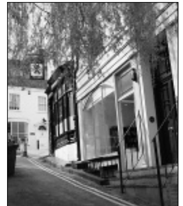
A view of the office from St Ann's Road
