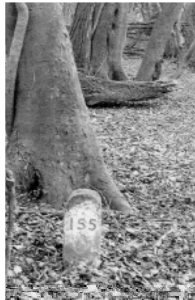
Marker stone over original pipeline
