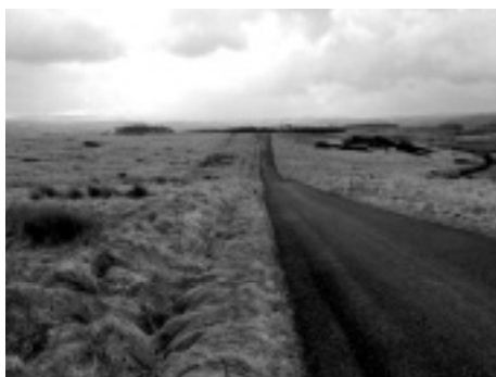
Roman Road Berm Ditches at Goat Gap, Yorkshire. Note the main roadside fosse (bottom, left of centre), and the left-hand Berm Ditch (far left), stretching away, parallel to the road. The right-hand (southern) berm ditch is nowadays less obvious.
